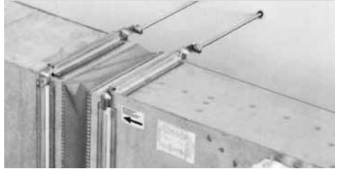
Figure 13 – Anchoring the fan
